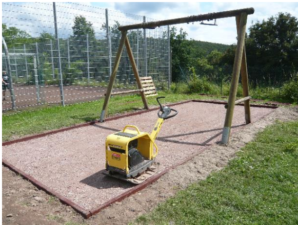
Crushed stones bed stable compacted
