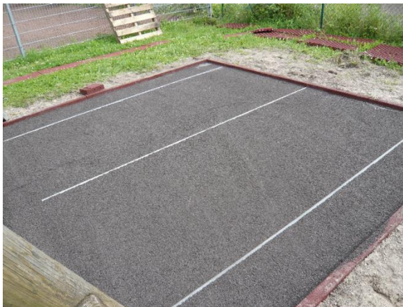
Levelling crushed sand/stone chippings
