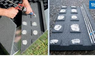
• The glue is laid on in circular form on the out-standing squares and along the rounded edge.
